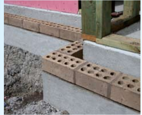
First course of brickwork laid with Termortar
