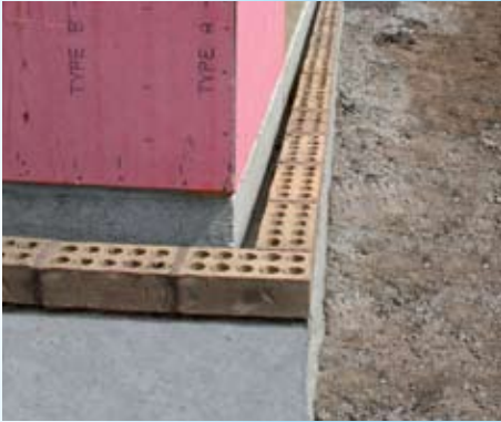
First course of brickwork laid with Termortar
